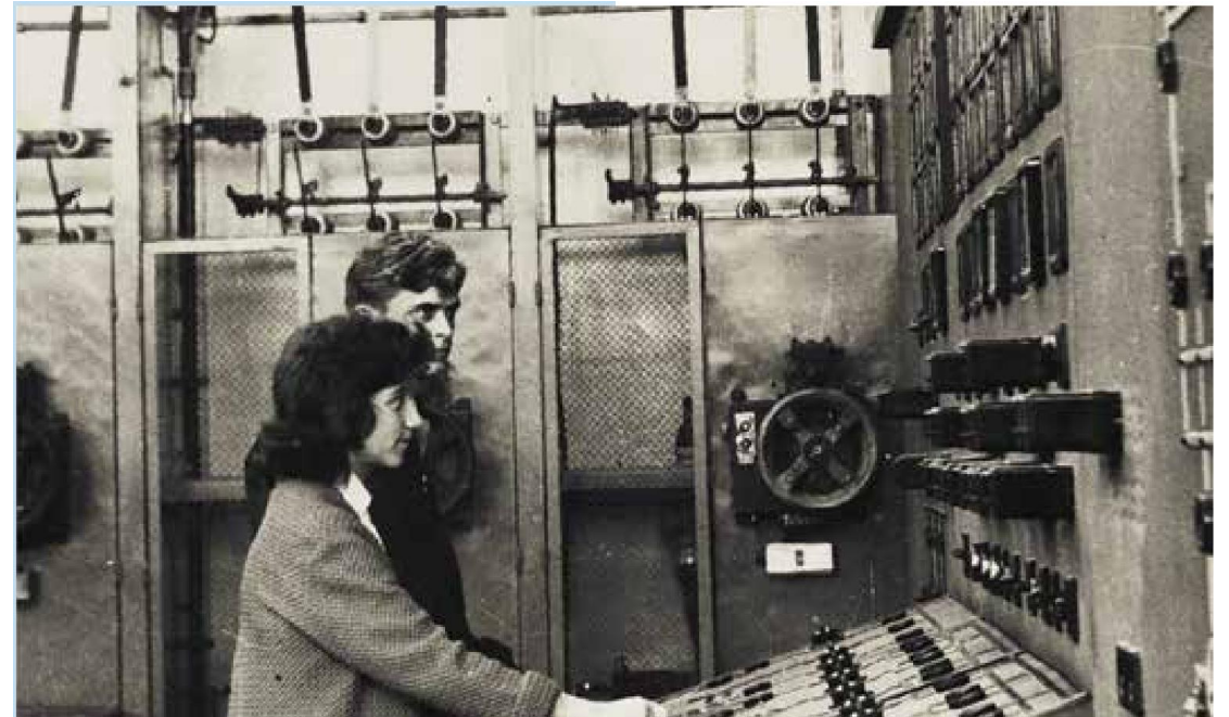
Laboratory of the Electrical Substations and Transformer Stations – Polizu campus
